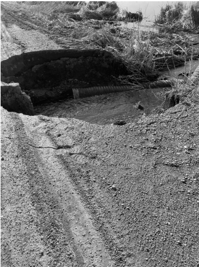
The above photo captures erosion and separated culvert (Good)
