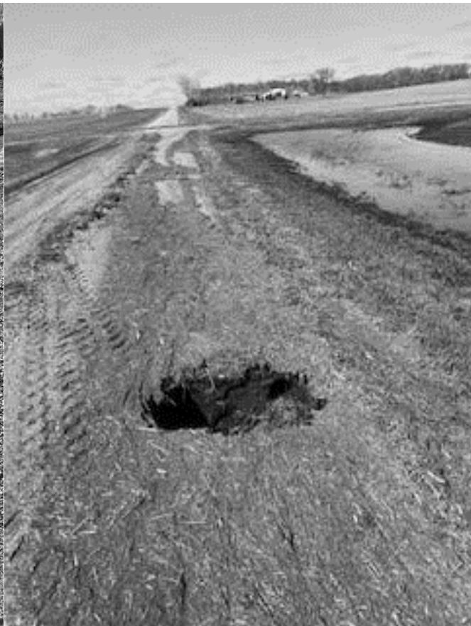
Photo identifies hole in the road. Damages Typical of a rusted culvert or animal damage (Poor and not eligible without additional photographic evidence Have the contractor take pictures of when repairing.
